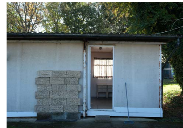
Prototype blocks stacked outside seasonal workers accommodation
