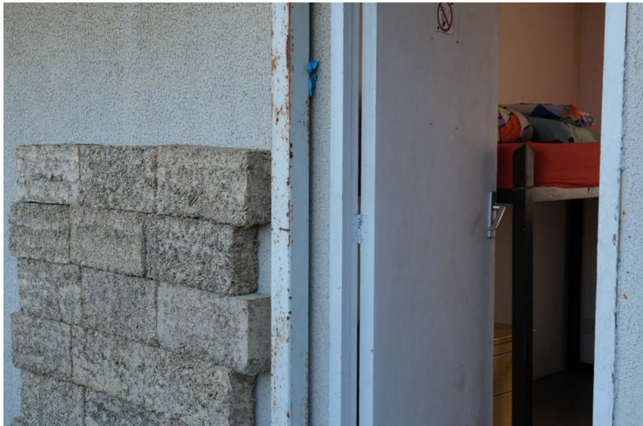
Prototype insulation block against facade of bunk houses
