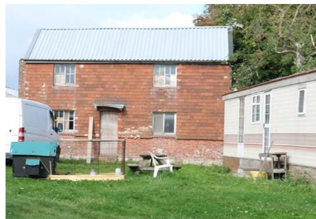
Farm buildings and worker's caravans in need of insulation
