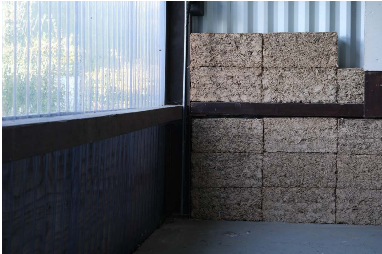
Prototype insulation blocks in farm workers common room
